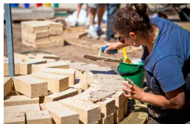
*Laying the Brikmakers clay bricks to create one of the 3m x 2m domes.*
